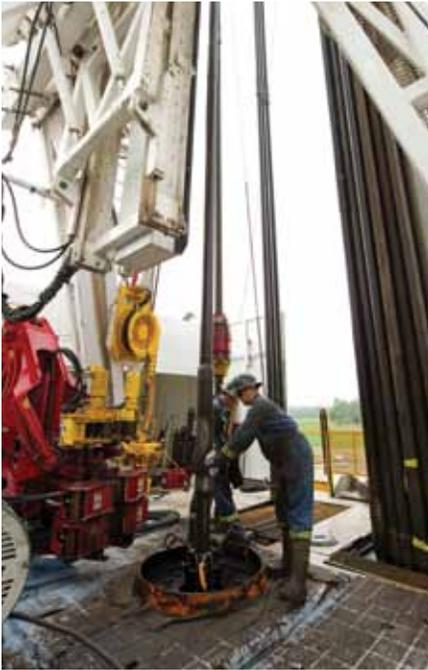
Drilling, casing and cementing procedures are designed to isolate the well from the potable groundwater zone.
